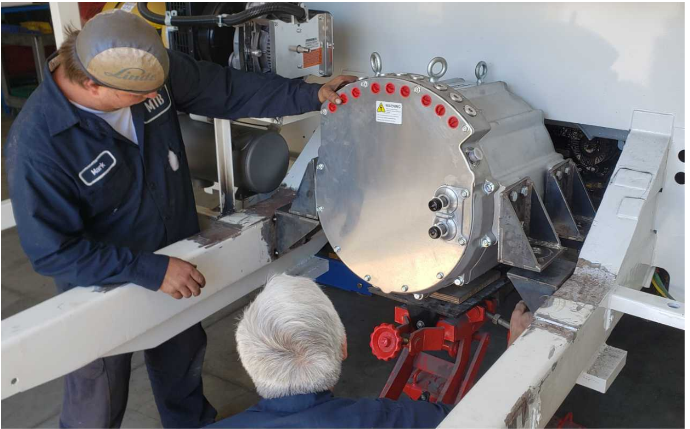
Work underway on MTB's demonstration bus conversion. Source: MTB Transit Solution
